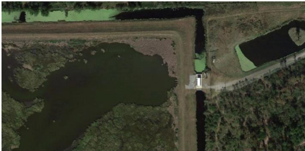
Figure 6. Satellite view of a stormwater pump station in the Terrebonne Basin
