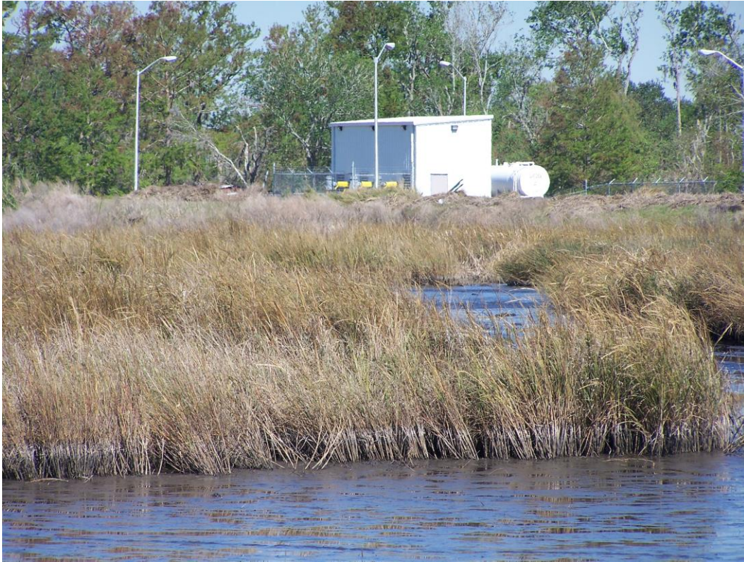
Figure 5. Image of a stormwater pump station within the Terrebonne Basin
